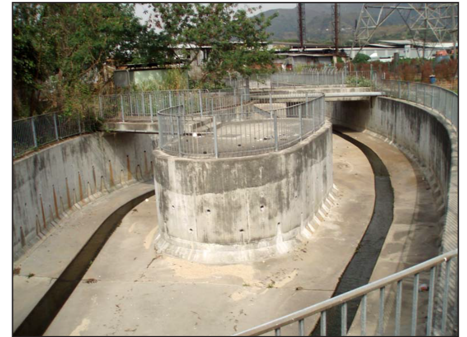
LR6 Drainage Channel
